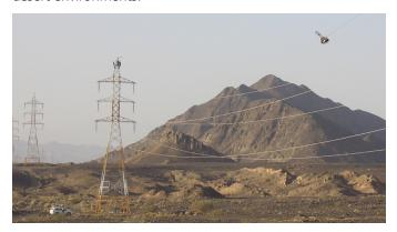
The installation technique is quick and has low impact on the surrounding environment and was installed on the ground wire under live line conditions. The lightweight equipment was able to be easily transported to towers over rocky uneven terrain.
