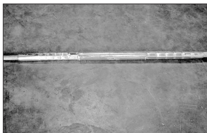
FIGURE 11c: Completed compression splice.
