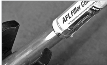
FIGURE 9: Inject AFC Filler Compound into the filler hole.
