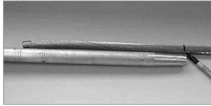
FIGURE 1: Mark the conductor and clean \frac{3}{4} the length of the aluminum body.
