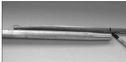
FIGURE 1: Mark the conductor and clean 1/2 the length of the sleeve.
