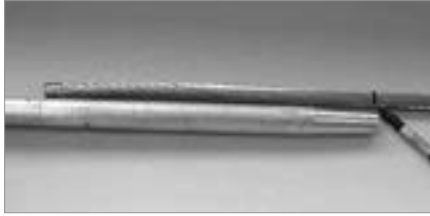
FIGURE 1: Mark the conductor and clean \frac{1}{2} the length of the sleeve.
