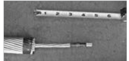
FIGURE 5a: Cut back the Aluminum strands on both conductors \frac{1}{2} the length of the Steel sleeve plus 1\frac{1}{2} inch (38.1 mm).
