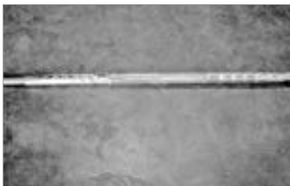
FIGURE 11c: Completed compression splice.
