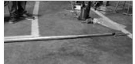
FIGURE 4: Slide sleeve over one conductor so it protrudes out the end.
