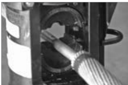
FIGURE 7a: Make the initial compression on center of Steel sleeve.
