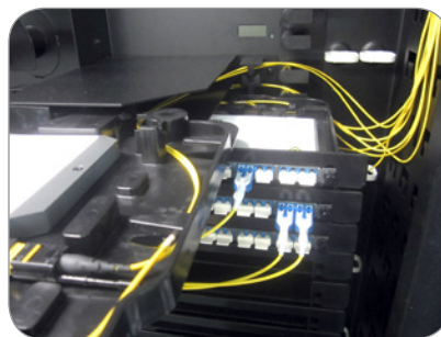
Figure 7. MTP leads connected to the cassette
