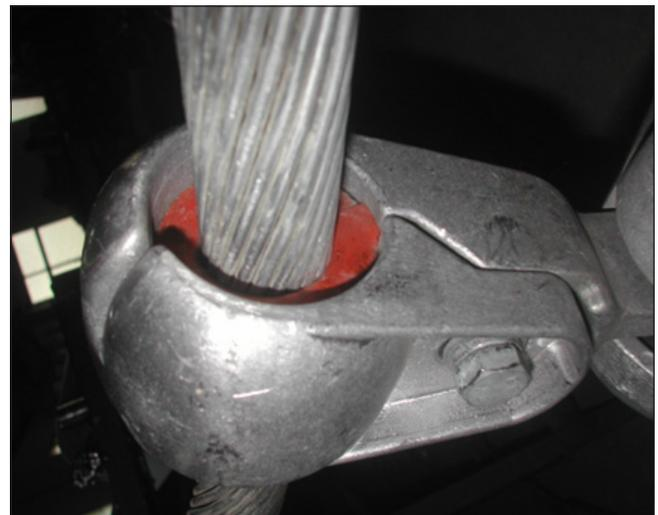
Each clamp of the Spacer Damper should look like this after installation.
