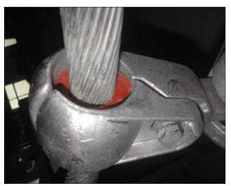
Each clamp of the Spacer Damper should look like this after installation.
