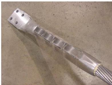
Filler Compound should be visible at end of the barrel during the final compressions (if adequate amount has been pumped in). Compressed portion of the Terminal Connector should have a smooth uniform appearance. Remove flash, if present, with file or emery cloth. Clean contact surface of Terminal Connector and Dead End pad.
