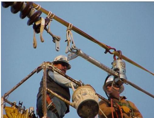
The photo to the left illustrates a setup, which works well to ensure a straight compression and easy maneuverability of the compressor. The conductor has been “tied off” to the tower with a sling and chain wrench. The compressor is then attached to the sling by a large shackle (the compressor is suspended upside down). The accessory and cable are tied to the sling ensuring all parts are straight and inline. The compressor can easily be slid along to each successive compression.
