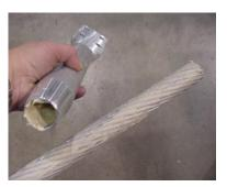
Inject sufficient filler compound in the end of the terminal bore and on the conductor to ensure that excess compound will be visible at terminal end when barrel is completely compressed.
