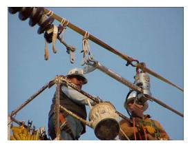
The photo to the left illustrates a setup, which works well to ensure a straight compression and easy maneuverability of the compressor. The conductor has been "tied off" to the tower with a sling and chain wench. The compressor is then attached to the sling by a large shackle (the compressor is suspended upside down). The accessory and cable are tied to the sling ensuring all parts are straight and inline. The compressor can easily be slid along to each successive compression.
