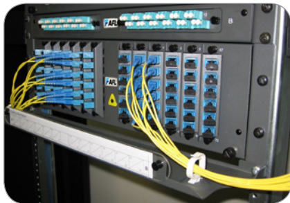
19" rail mounted cable tray fixed beneath enclosure
