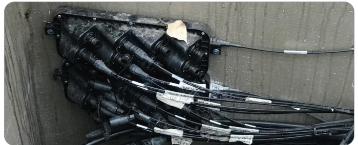
Figure 4 — Handhole Mount Application
