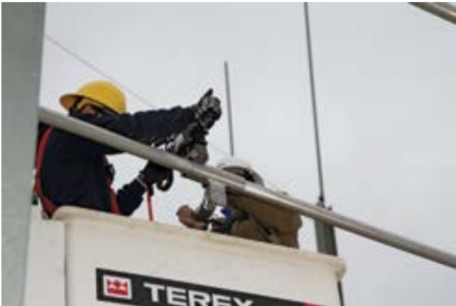
After using the Swage gauge to mark insert depth, the Swage Press and Die Set compress the Bus Tee fitting onto the pipe.
