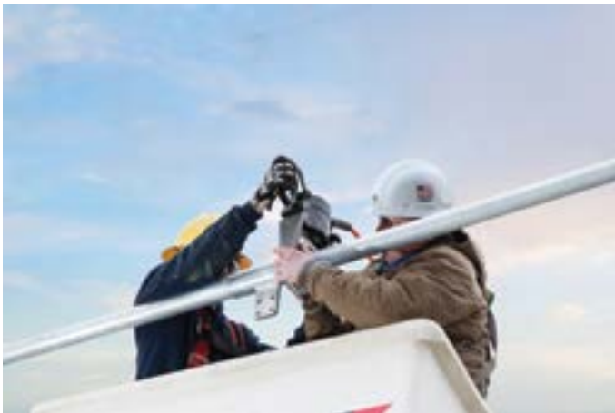
Installing a Swage Tee fitting in South Carolina.
