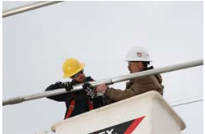
Fit the Bus Tees the pipe. The fitting comes apart for ease of installation.
