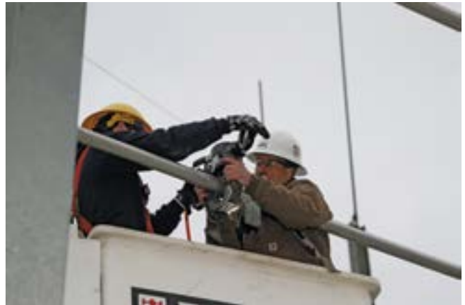
After using the Swage gauge to mark insert depth, the Swage Press and Die Set compress the Bus Tee fitting onto the pipe.
