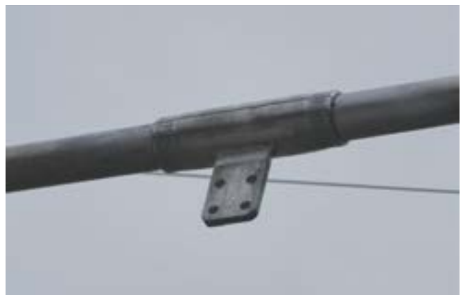
The finished Swage Bus Tee fitting
