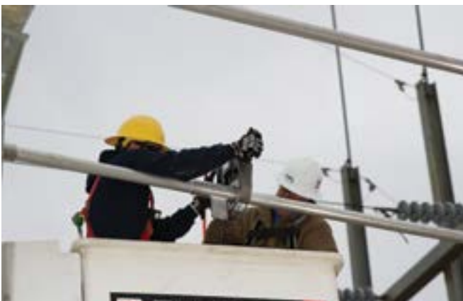
Compressing the fitting
