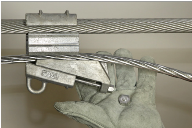
Breakaway bolt head sheared off.
