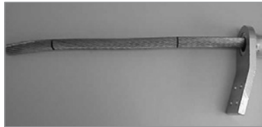
FIGURE 3: Slide aluminum dead end body over conductor.
