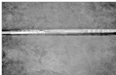
FIGURE 11c: Completed compression splice.
