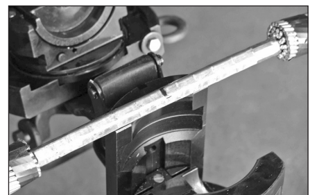
FIGURE 7b: Overlap each compression on Steel sleeve \frac{1}{4} inch (6.4 mm).
