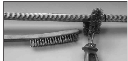
FIGURE 2: Clean the outer strands of the conductor with a wire brush.
