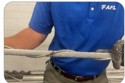
Figure 3 — Aligning first inner rod
