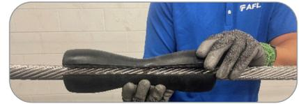
Figure 5 — Aligning insert halves
