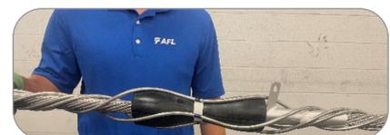
Figure 8 — Four outer rods installed
