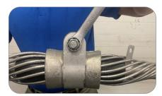
Figure 11 — Tightening bolt with wrench
