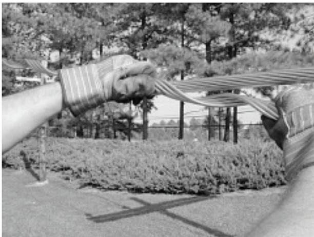
3. Place the center of the first subset onto the conductor and begin wrapping.
