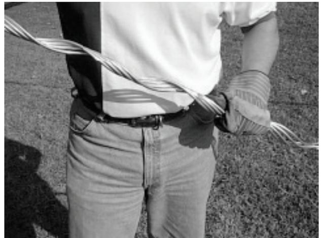
2. Continue twisting the rods until they are completely subsetted end to end. Repeat the procedure until all the rods are in subsets.
