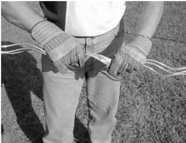
1. For conductor sizes 4/0 and above, a maximum of 4 rods may be subsetted together. To subset, hold the rods flat making sure none of the rods are crossed, then twist the rods with the lay direction until they subset together. For sizes less than 4/0 see General Notes on back.
