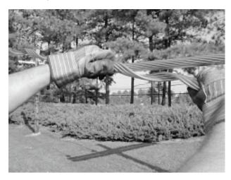
3. Place the center of the first subset onto the conductor and begin wrapping.
