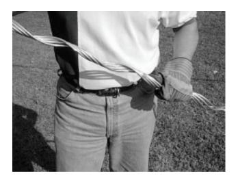
2. Continue twisting the rods until they are completely subsetted end to end. Repeat the procedure until all the rods are in subsets.
