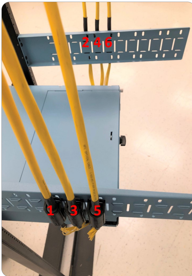
Figure 10. Recommended Trunk Cable Installation Order
