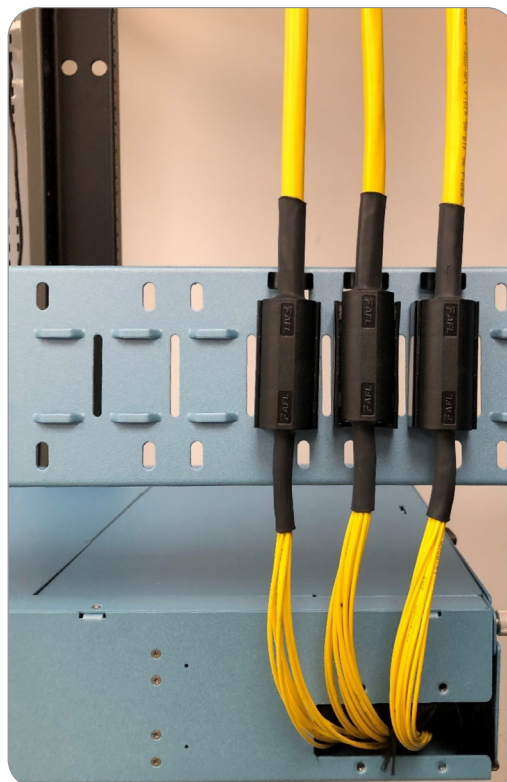
Figure 9. Cable Entrance Alignment
