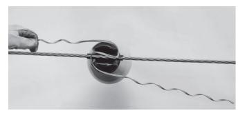
**3.** Rotate the Distribution Tie counter clockwise ensuring both legs cross under the conductor.
