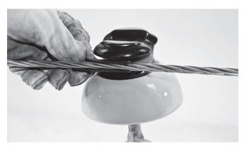
**2.** Position the midpoint of each pad slightly beyond center of the insulator groove making the span between each Tie Pad larger.
