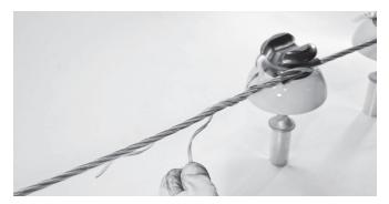
**6.** Lift up the leg and wrap it around the conductor. Ensure the Distribution Tie end fully snaps into place. This may require more pressure than the pressure to wrap.
