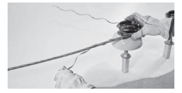
**5.** Wrap the second leg around the insulator passing the first leg, so it crosses at one of the marks.
