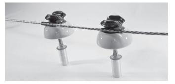
**3.** Install the Double Side Tie around the neck of the insulator. Ensure the leg of the tie with the crossover marking is on the same side as the conductor. Pull the tie snug against the insulator neck so that it will be properly seated.
