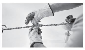
**7.** One side is now complete. Repeat steps 3-6 to the other side with the second tie. (Note: Wrap the tie over the pad in this installation.)
