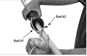
FIGURE 3: Installing the second armor rod
