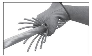
FIGURE 6: Wrapping the ends of the rods
