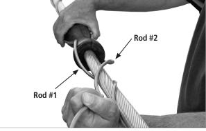
FIGURE 3: Installing the second armor rod
