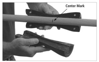
FIGURE 2: Center insert on mark
