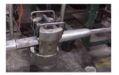
Make initial compression on either side of Joint starting at the "Start" knurl. Make the second compression on the opposite end of the joint at the other "Start" knurl. Continue making compressions to the end of the joint. **Overlap each successive compression by approximately 0.50 inch** (1.27 cm). Do not "skip bite." Complete die closure is required for each compression. Go back and complete the compressions on the opposite end. The center portion of the Joint is not compressed.
