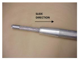
Slide aluminum body over the conductor and beyond mark until sufficient working length protrudes from barrel end. Straightening the conductor as much as possible will also aid in this installation step.
