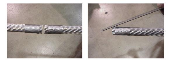
Straighten several feet of the conductor removing the set caused by the reel.
