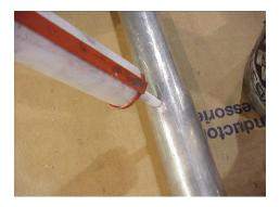
Inject AFL Filler Compound into filler hole. AFL will specify amount needed base on accessory being used. Insert, then drive filler plug into hole and peen edge of hold over top surface of plug.
