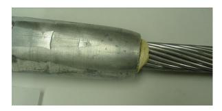
Filler Compound should be visible at end of the barrel during the final compressions (if adequate amount has been pumped in).
