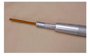
**NOTE:** It is extremely important not to nick the core during cutting back of the aluminum strands. If this is done, the ultimate strength of the Joint will be reduced.
