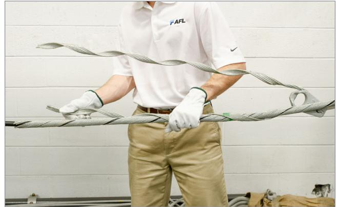
8. Split the legs to ease application and apply them completely. Make sure all rod ends are snapped into place.
