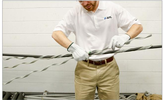
5. Split rod ends and apply them completely. Make sure all rod ends are snapped into place.
