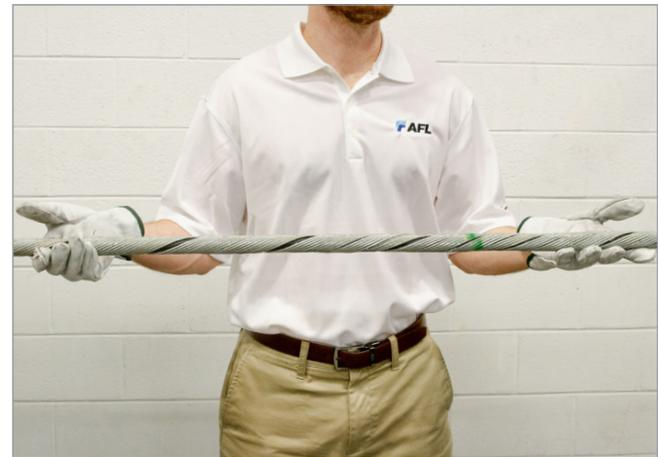
6. Insert the dead end loop through the thimble clevis provided (or a similar attachment hardware). Align the crossover mark of the dead end with the color code mark of the structural reinforcing rods.
