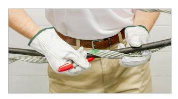
2. Notice that the color mark of the Structural Reinforced Rods is offset from the center (the length from one end of the subset to the mark is shorter than the other). With the short length positioned near the structure, align the color code mark to the reference mark you just made and apply the first subset.
