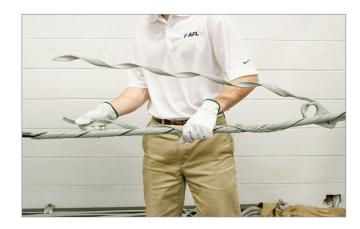
**8.** Split the legs to ease application and apply them completely. Make sure all rod ends are snapped into place.
