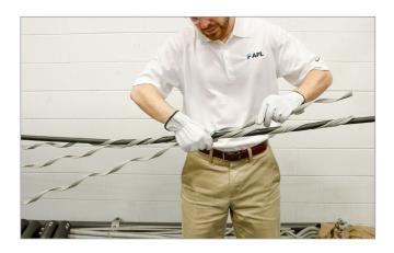
**5.** Split rod ends and apply them completely. Make sure all rod ends are snapped into place.
