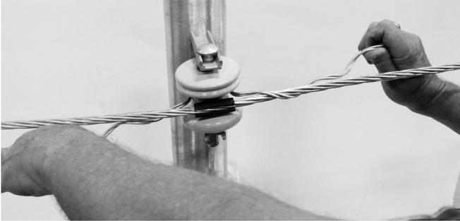
6. Finish by fully wrapping both legs around the conductor. Ensure the Quick Spool Tie end fully snaps into place. This may require more pressure than the pressure to wrap.
