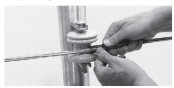
**2.** Ensure the Tie Pad is protecting the conductor from coming in direct contact with the insulator.
