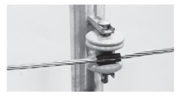
**3.** Install the Easy Tie by feeding one tie leg behind the spool. Then pull the tie leg under the conductor while keeping the right tie leg over the conductor.
