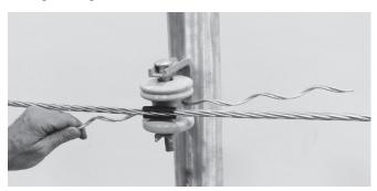
**4.** Position the Quick Spool Tie around the neck of the insulator. Be sure the conductor is between the two legs of the Easy Tie. (left tie leg below, right tie leg above conductor)
