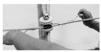
6. Finish by fully wrapping both legs around the conductor. Ensure the Quick Spool Tie end fully snaps into place. This may require more pressure than the pressure to wrap.
