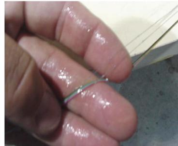
**11.5** Repeat steps 10.3 through 10.4 on each of the fiber bundles. Separate each group of bundled fibers to assure easy identification (see Fig. 27).
