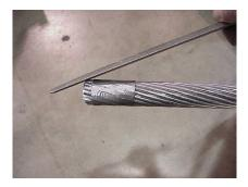
Prior to cutting, wrap tape around the conductor to help maintain the round contour, making it easier to slide the end through the aluminum dead end. File approximately 0.09 inch chamfer on the end of the conductor. (The larger the chamfer, the easier the conductor will slide through).
