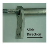
Slide aluminum dead end body (barrel first) over the conductor until sufficient working length protrudes from tongue end.
