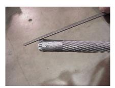
Prior to cutting, wrap tape around the conductor to help maintain the round contour, making it easier to slide the end through the aluminum dead end. File approximately 0.09 inch chamfer on the end of the conductor. (The larger the chamfer, the easier the conductor will slide through).
