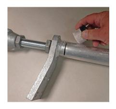
Make initial compression on the dead end body over the steel threads beginning at the start knurl near the tongue. Continue making compressions overlapping the previous compression by approximately 0.50 inch. Complete die closure is required for each compression. Continue compressing to end of dead end barrel.
