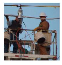
**Setup 2:** The compressor sits on a board, which sits on the rails of the high lift. The board and compressor can be slid along to each successive compression. The accessory and cable must be supported and all parts must be straight and in-line or bowing will occur.
