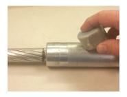
Lubricate outside surface of joint with "Accu-Lube" or similar lubricant, or cover barrel with accessory plastic wrapper.
