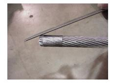
Prior to cutting, wrap tape around the conductor to help maintain the round contour, making it easier to slide the end through the aluminum joint. File approximately 0.09 inch chamfer on the end of the conductor. (The larger the chamfer, the easier the conductor will slide through).
