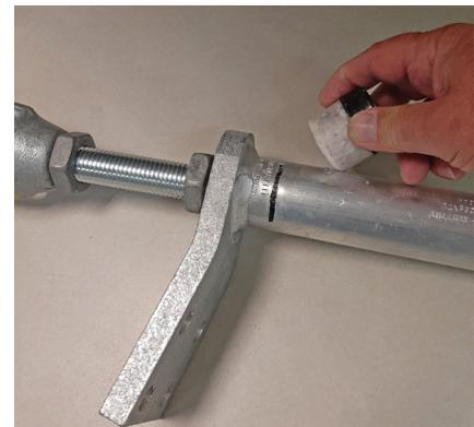
Make initial compression on the dead end body over the steel threads beginning at the start knurl near the tongue. Continue making compressions overlapping the previous compression by approximately 0.50 inch. Complete die closure is required for each compression. Continue compressing to end of dead end barrel.
