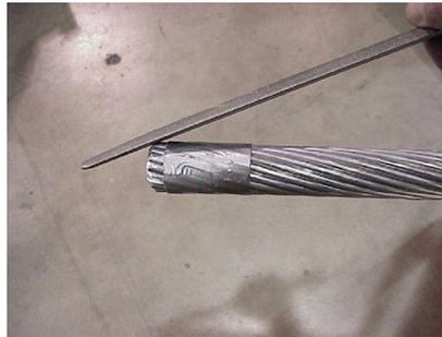
Prior to cutting, wrap tape around the conductor to help maintain the round contour, making it easier to slide the end through the aluminum joint. File approximately 0.09 inch chamfer on the end of the conductor. (The larger the chamfer, the easier the conductor will slide through).
