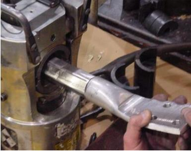
Press the Terminal Connector over the conductor. Make the initial compression at the start knurl. Continue making compressions to the end of the Terminal Connector barrel, overlapping the previous compression by approximately 0.50 inches. Complete die closure is required for each compression.
