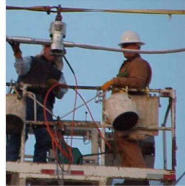
**Setup 2:** The compressor sits on a board, which sits on the rails of the high lift. The board and compressor can be slid along to each successive compression. The accessory and cable must be supported and all parts must be straight and in-line or bowing will occur.
