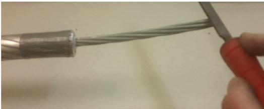
File chamfer on end of core and end of aluminum strands to remove burrs and sharp edge. Chamfer will reduce the expanded diameter of the core (due to cutting) and ease the installation of the adjustable clevis/"core grip".
