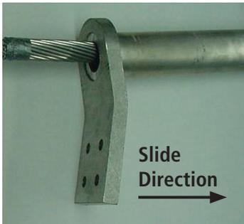
Slide aluminum dead end body (barrel first) over the conductor until sufficient working length protrudes from tongue end.
