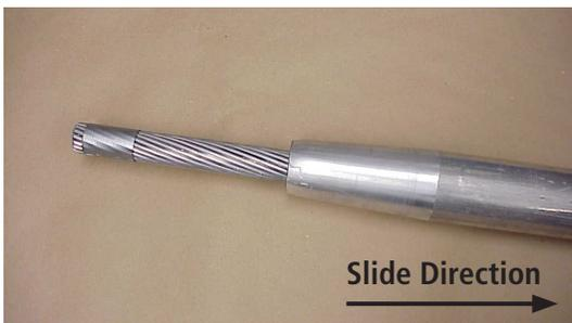
Slide aluminum body over the conductor and beyond mark until sufficient working length protrudes from barrel end.
