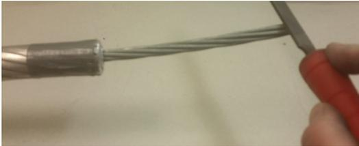
File chamfer on end of core to remove burrs and sharp edge. Chamfer will reduce the expanded diameter of the core (due to cutting) and ease the installation of the Steel Eye/"Core Grip".
