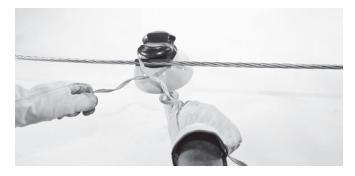
**6.** Finish fully wrapping both legs around the conductor. Ensure the Side Tie end fully snaps into place. This may require more pressure than the pressure to wrap.
