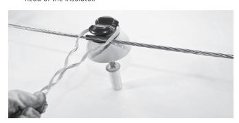
**4.** Position the Side Tie around the neck of the insulator. Be sure the conductor is between the two legs of the Side Tie.
