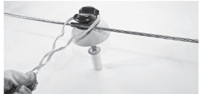
4. Position the Side Tie around the neck of the insulator. Be sure the conductor is between the two legs of the Side Tie.
