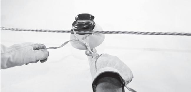
6. Finish fully wrapping both legs around the conductor. Ensure the Side Tie end fully snaps into place. This may require more pressure than the pressure to wrap.
