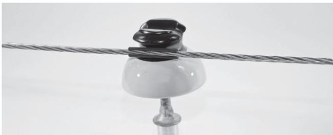
3. Install the Side Tie over the pad by squeezing the two Tie legs. The loop will enlarge enabling enough space to slide over the head of the insulator.
