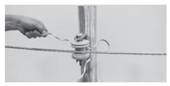
2. Position the Spool Tie around the neck of the insulator. Be sure the conductor is between the two legs of the Spool Tie. (left tie leg above, right tie leg below conductor)
