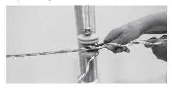
**4.** Ensure the Tie Pad is protecting the conductor from coming in direct contact with the insulator.
