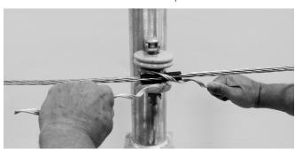
**6.** Finish fully wrapping both legs around the conductor. Ensure the Spool Tie end fully snaps into place. This may require more pressure than the pressure to wrap.
