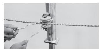
**3.** Apply the Tie Pads to the conductor so the conductor does not come into direct contact with the insulator. Keep the tie pad slit facing outward.
