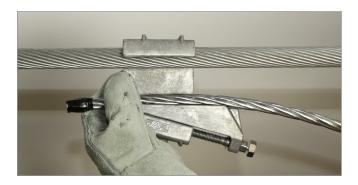
**NOTE:** Each interface is stamped with "Tap" and "Run" as well as the most common conductor size in the range. Ensure that the interface is in the correct orientation prior to installing.
