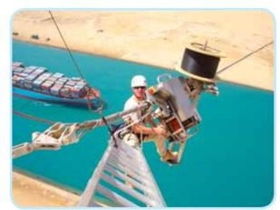
There were aircraft warning spheres on the line which had to be removed using a specially adapted trolley to safely support two men as they worked 200 m above the Canal. A novel fixture system was designed to load the wrapping machines 4 m out on the line ready to start spinning.
