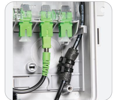
**Figure 12** – Attach foam and tiewrap to secure premise drops
