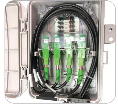
**Figure 11** – Clean and install premise drop connector
