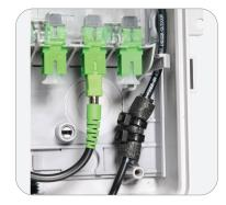
Figure 12 – Attach foam and tiewrap to secure premise drops
