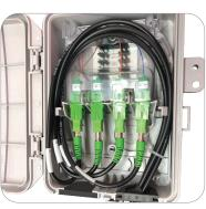
Figure 11 – Clean and install premise drop connector
