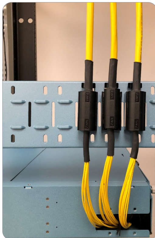
Figure 9. Cable Entrance Alignment
