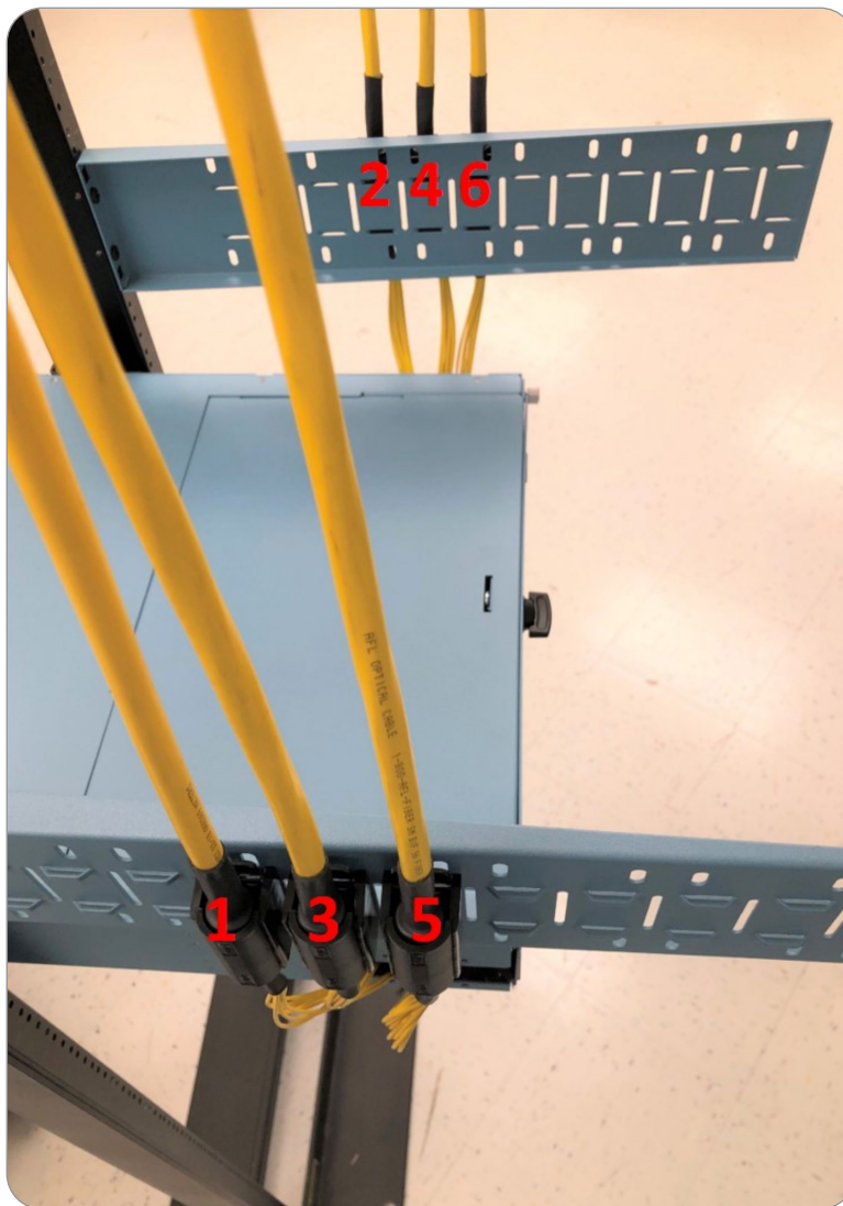
Figure 10. Recommended Trunk Cable Installation Order
