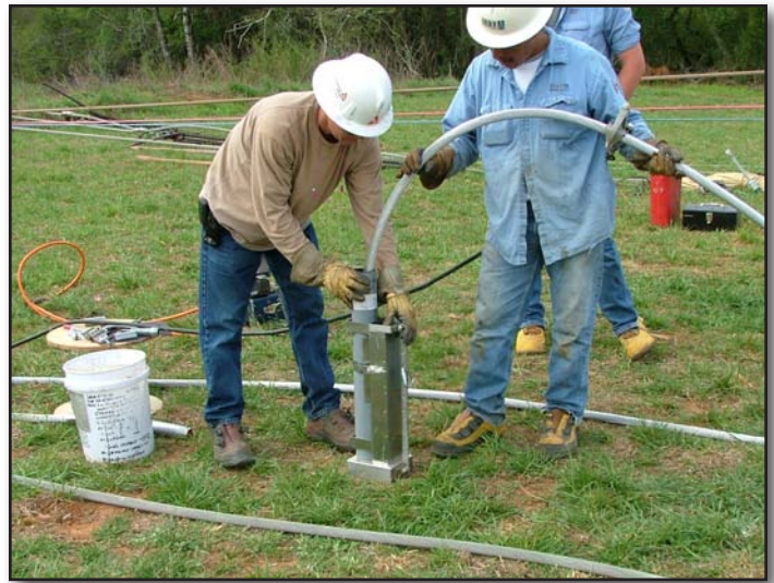
GPC and contract crews cleaning the conductor using the conductor cleaner.
