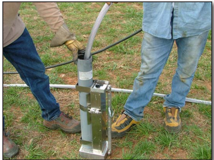
Close up of conductor cleaner in action.
