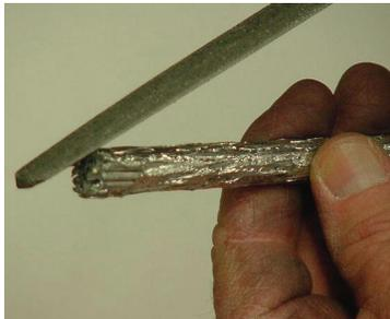
Insert conductor's core into steel forging. Ensure distance from the end of barrel to aluminum strands is 1.50 inches.
