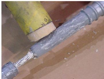
Core must be straight as it enters bore. Support conductor while compressing to ensure a straight compression.
