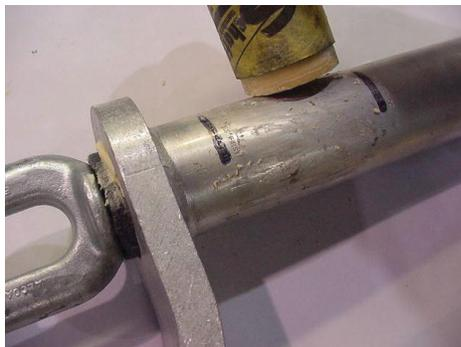
Make initial compression on the dead end body over the steel shank beginning at the "Start" knurl nearest the dead end tongue. Continue making compressions to the "Stop" knurl, overlapping the previous compression by approximately .50 inch. Complete die closure is required for each compression (see Fig. 14).
