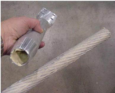
Insert conductor end into terminal barrel to the mark on the conductor.
